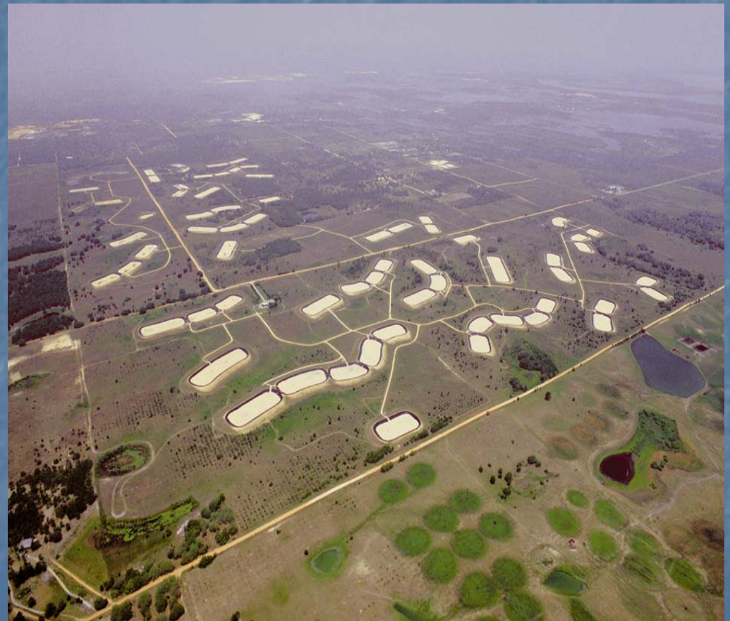
Rapid infiltration basins. (Photograph courtesy of Water Conserv II facility, Orlando, Florida.)
