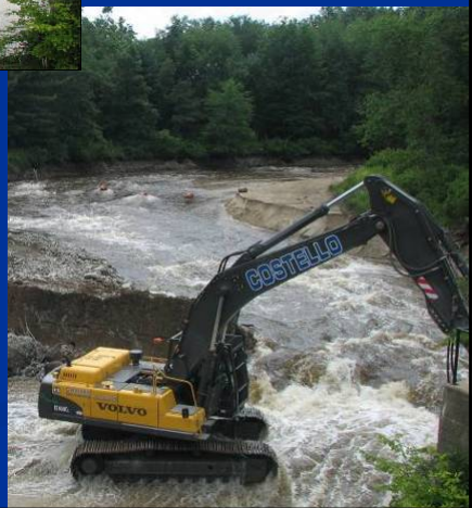
Merrimack Village Dam Souhegan River Merrimack, NH
