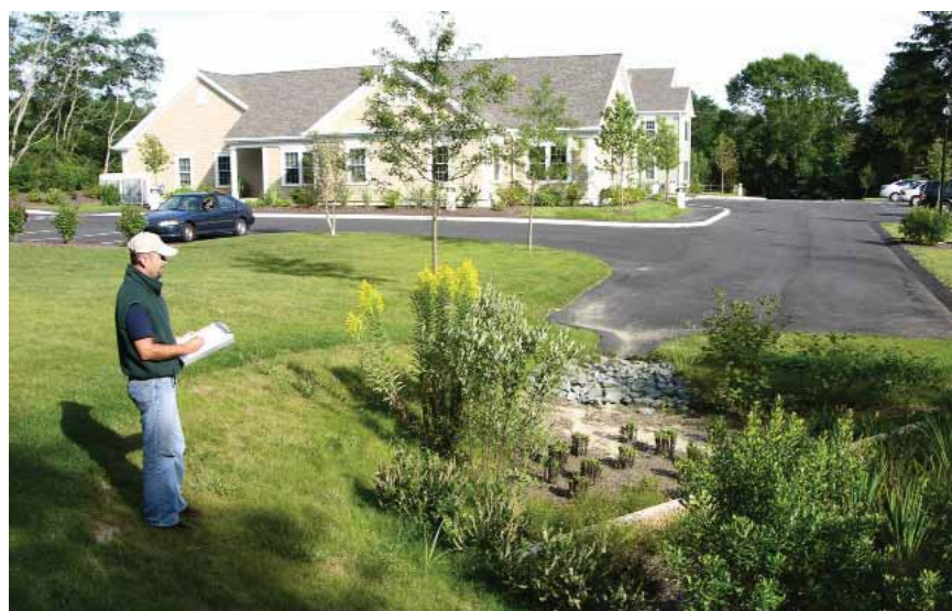
Figure 9-6 Inspection of Bioretention Facility.
