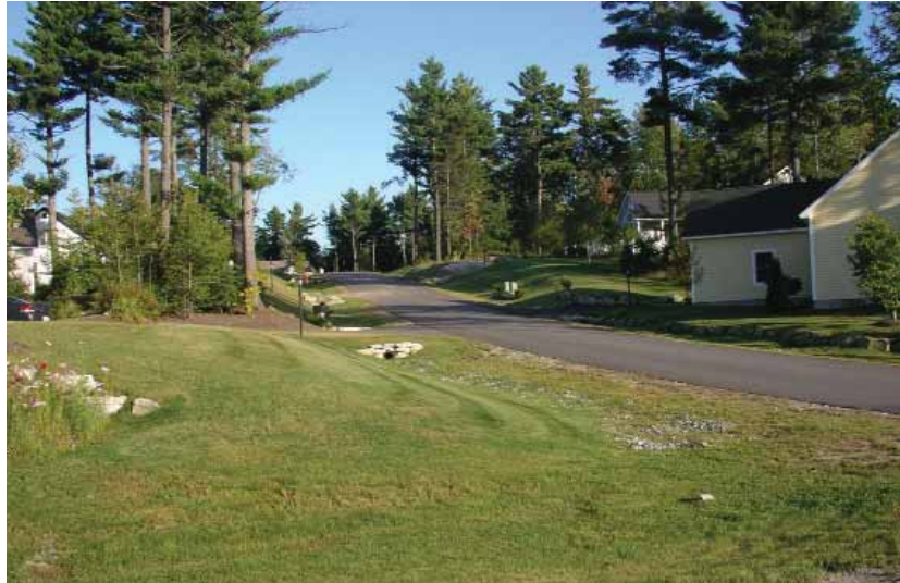
Vegetated swales are used to manage runoff from adjacent roads instead of having typical “curb and gutter” systems. (HW photo)
