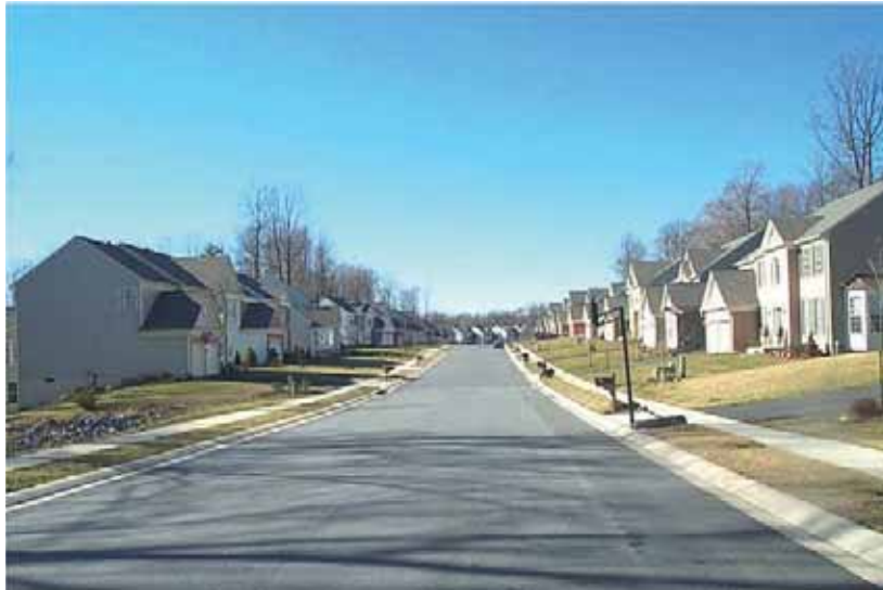
Figure 5-1 Excessive Roadway Design.
