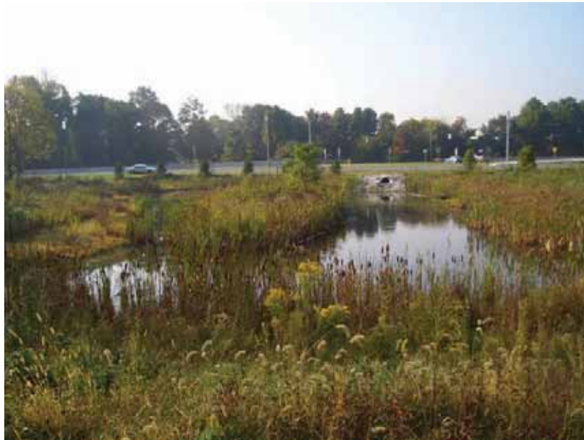
Figure 9-9 Stormwater Facility Requiring Regular Inspection.
