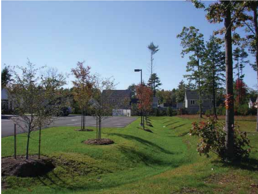
Figure 1-3 Vegetated Swale Designed to Treat Stormwater Runoff.
