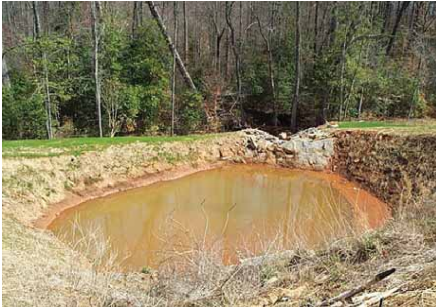
Figure 9-4 Properly Installed Erosion and Sediment Control Practice.
