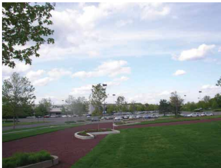
Regular parking areas are constructed with asphalt (background) while overflow areas show pervious travel lanes and reinforced turf in the foreground of this photo. (HW photo)
