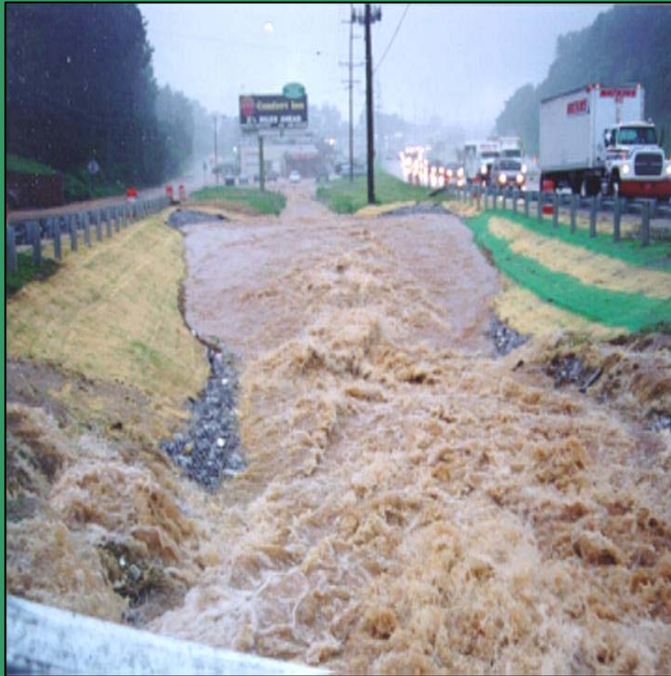
More Frequent Flooding
