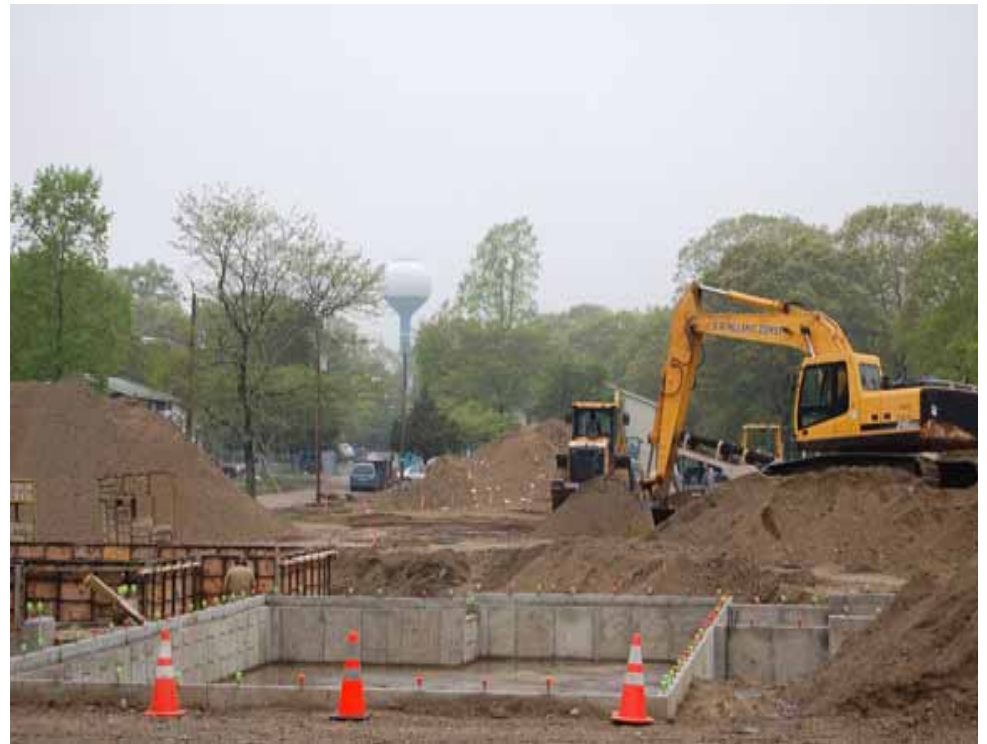
Construction at Kingstown Crossings, supported through BHRI
