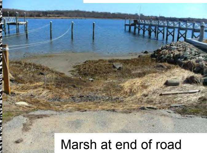
Road removal area
