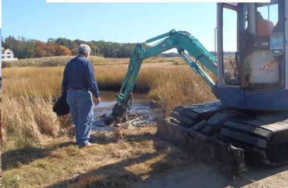
Clearing clogged culvert
