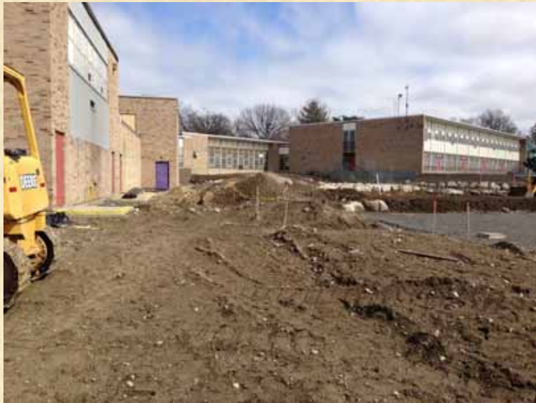
Ballfield & Water Park Under Construction
