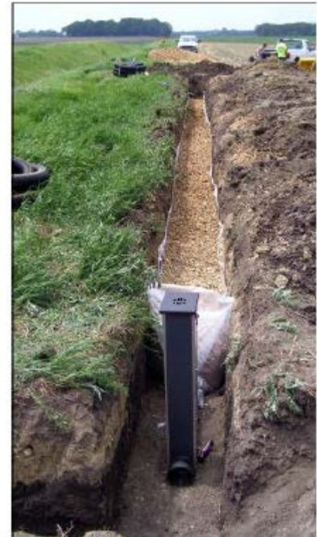
View of Bioreactor installation along field edge. Source: photo Marc Dittrich, Minnesota Dept. of Ag.
