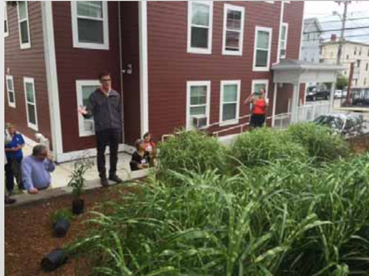
Affordable Housing units with GI landscaping and parking area on Manton Avenue in Providence
