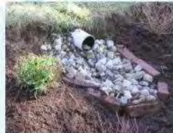
Solution Weed as needed and remove sediment and other debris. Look for bare soil in the area draining to rain garden and correct the problem at the source. Above is a typical rain garden inlet. The stone and pipe will need cleaning out from time to time.
