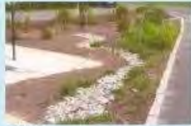
Solution Add river rock and more plants to better dissipate the flow of water.
