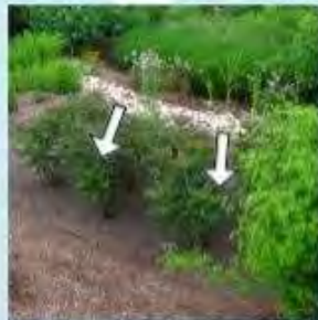
Problem The lowest points in the rain garden have begun to gather dark sediment build-up over the brighter mulch layer.
