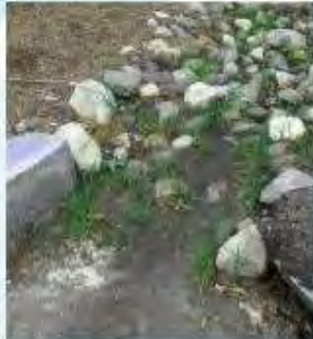
Problem There is sediment build-ups in the inlet, covering the river rock, allowing plants to take root, and blocking flow into the garden.
