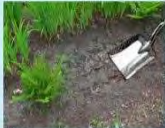
Solution Carefully remove top layer of sediment with a flat shovel to prevent or stop clogging. Add fresh mulch if needed.
